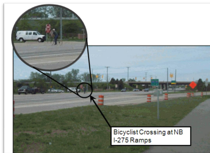
Figure 4.5 – Bicyclist Crossing M-153 east of the NB I-275 Exit Ramp Intersection
