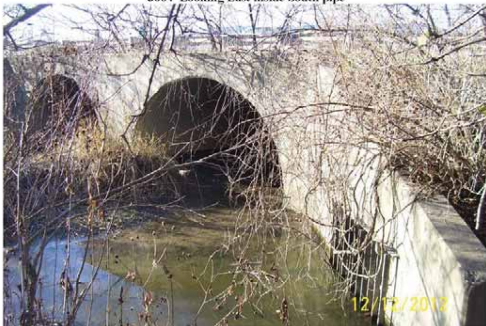
3605 East end of pipes
