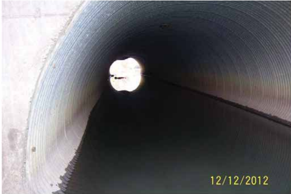
3604 Looking East inside South pipe
