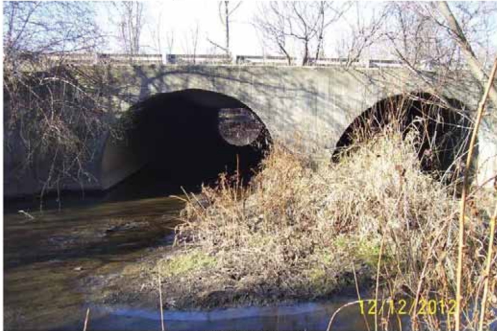
3608 East end of pipes
