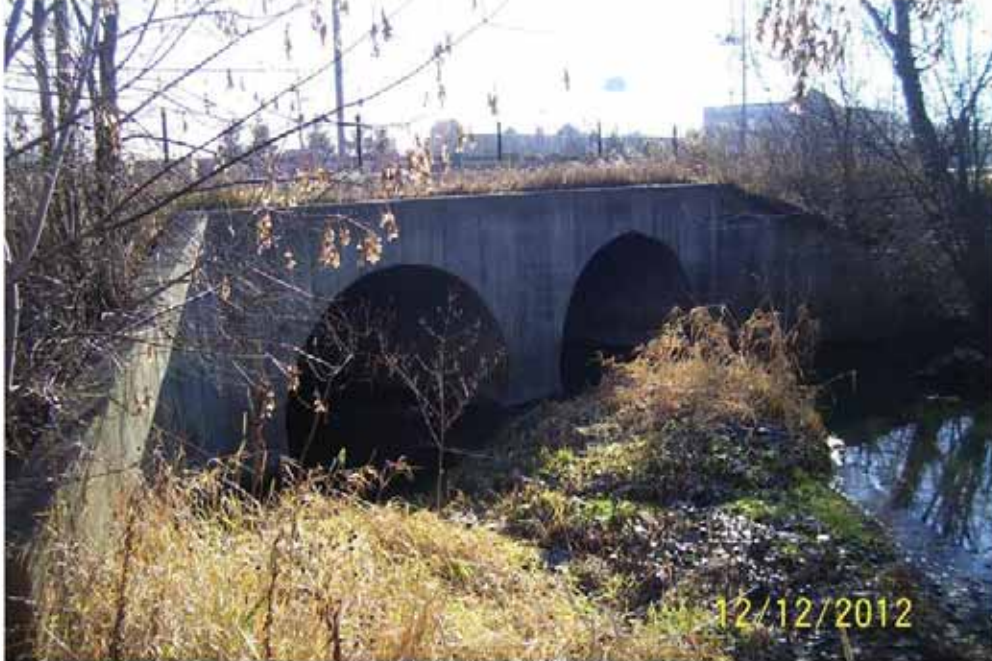
3602 West end of pipes
