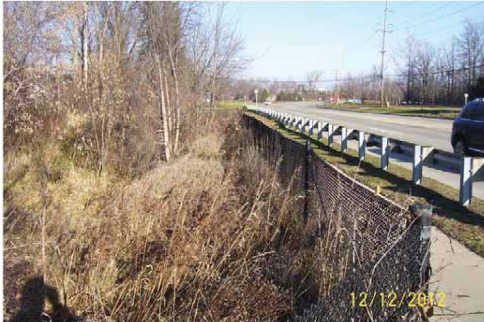
3600 Looking North, West end of culverts
