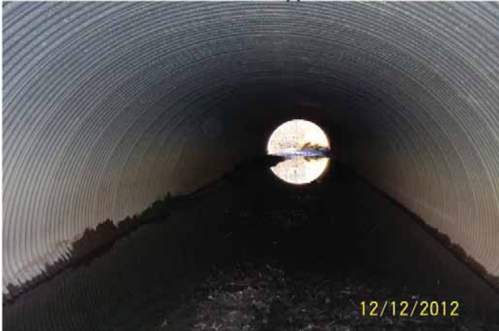
3603 Looking East inside North pipe
