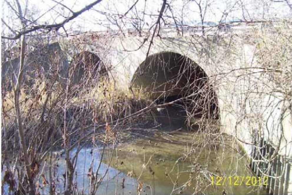
3606 East end of pipes
