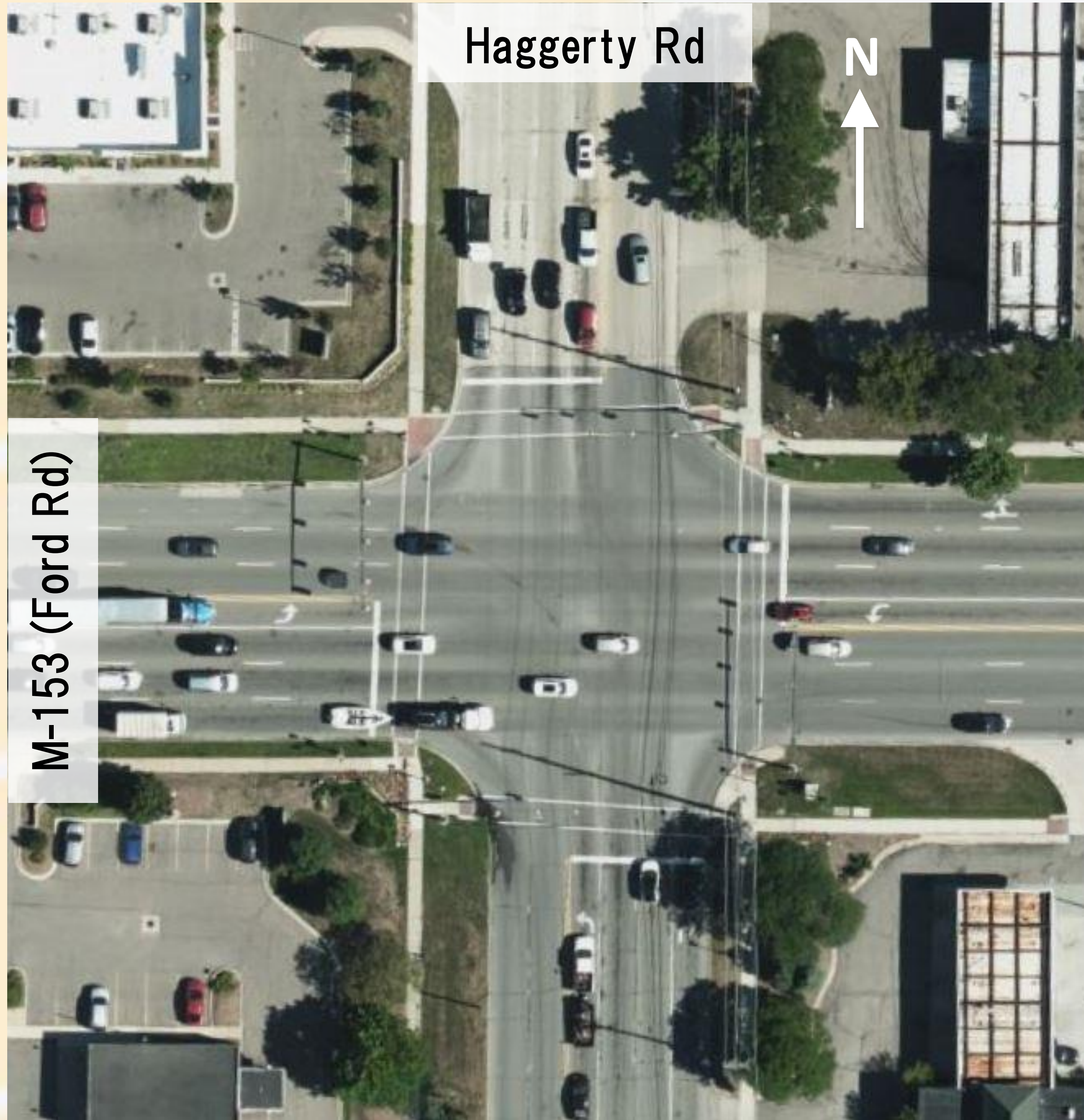
Current M-153 (Ford Road)/ Haggerty Road intersection
